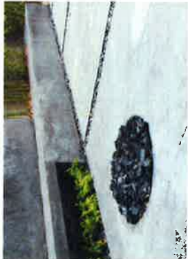
INSITU CONCRETE PAVING & SEATING EXTRUSIONS
